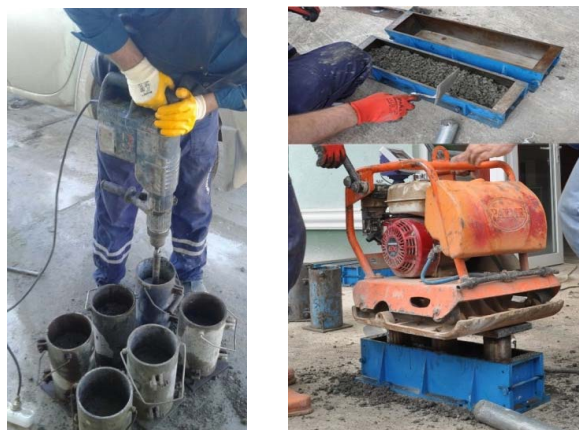
Figure 3. The Vibrating hammer (a), The Vibratory soil plate compactor (b)
