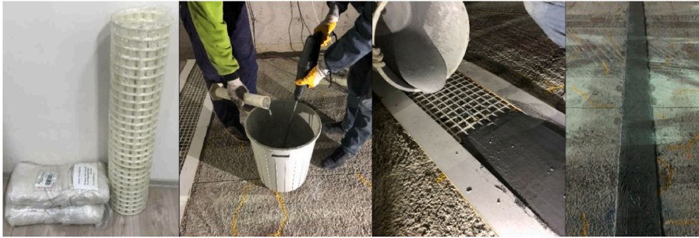
Fig. 5. Fiberglass geogrid and grout mortar application on contraction joint.
