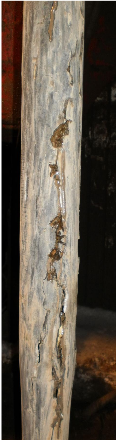
Fig. 6. Cracks and fractures in the drill pipe after torpedoing
