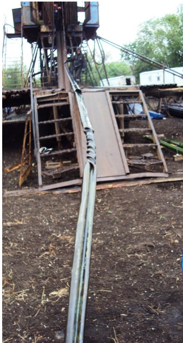
Fig. 2. Drilling tool extracted from the well
